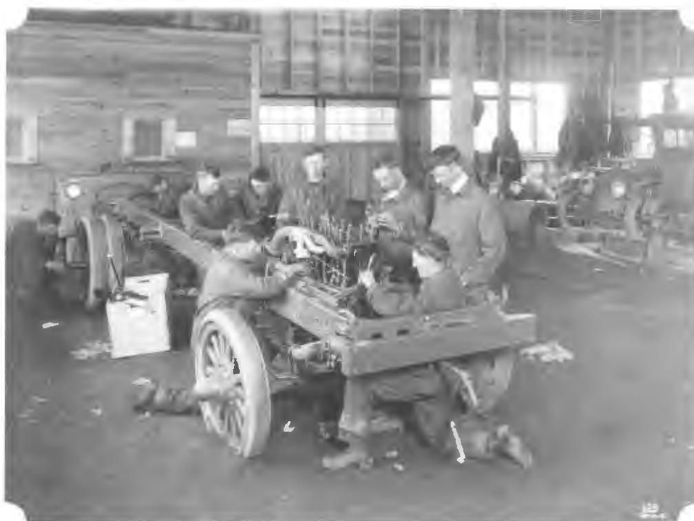
Engine repair on a Liberty Truck, May 1918 (University of Pittsburgh)
